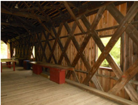
Figure 5: The Major A. Frederick Oberline Bridge showing a lattice design.
