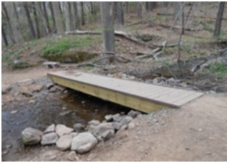
Figure 1: The above beam bridge is on a trail in a park in Branford, CT and is a cross over a small stream. The sketch shows a straight bridge between two land pieces. The dashed lines show that weight on the bridge will cause it to sag and with too much weight the bridge will collapse.
