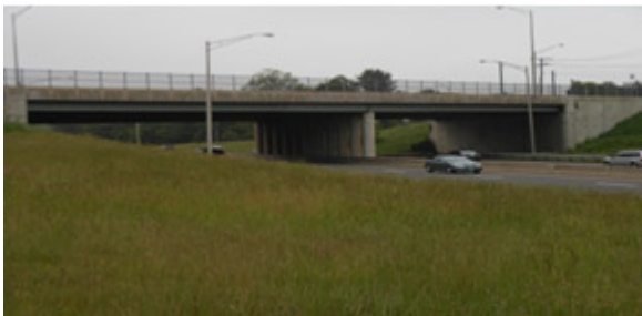
Figure 2: Pictured is a compression bridge on an interstate highway in Branford, CT. In the sketch, the arrows show where the compression forces act on the bridge. Compression is a pushing force. In this case, the concrete piling pushes down to the ground and the ground pushes up to the piling. Likewise, on the bridge, the two forces push against each other at the piling. Notice that the tension is halved.
